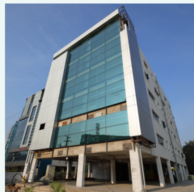
Location: LB Nagar Established: 2016 Bed Capacity: 100
